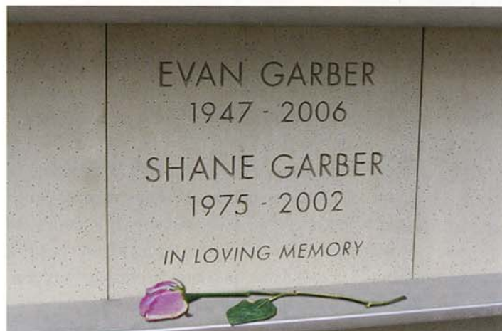
A set font style and size of sandblasted inscriptions on columbaria niche shutters creates consistency among interments units.
